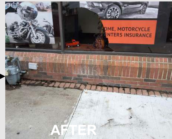
Broken Glass Clean Up
