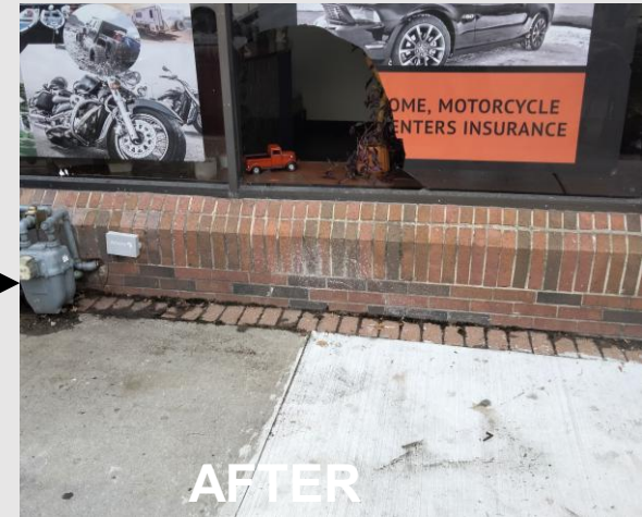
Broken Glass Picked Up
