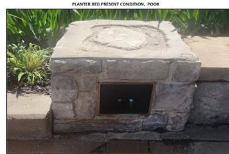
PIAC PROJECT OBJECTIVE—REPLACE MISSING CONCRETE TOPS, MORTAR AS NEEDED
